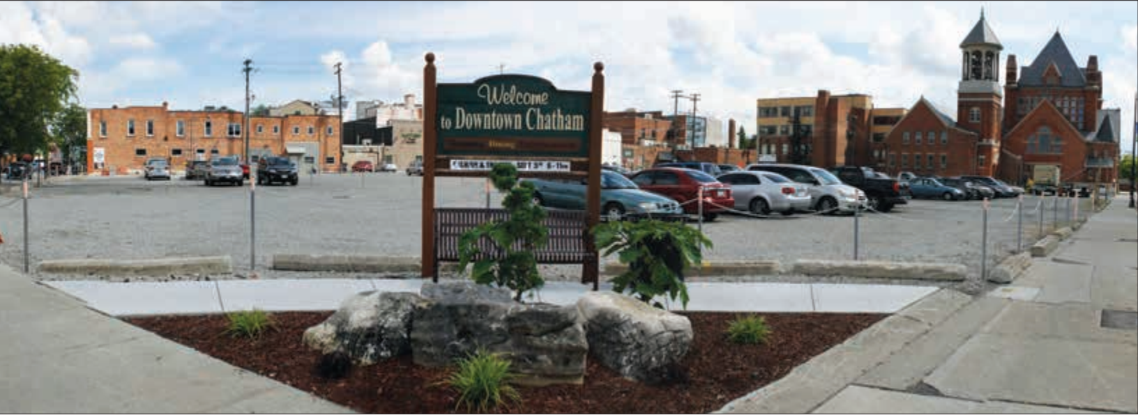
Image below: Wellington & Fourth Street, Parking Lot Resurfacing, and a newly landscaped corner with downtown gateway sign.
